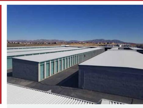
The Store America facility in Victorville, CA was leaking from seams and missing screws. These issues required constant maintenance.
